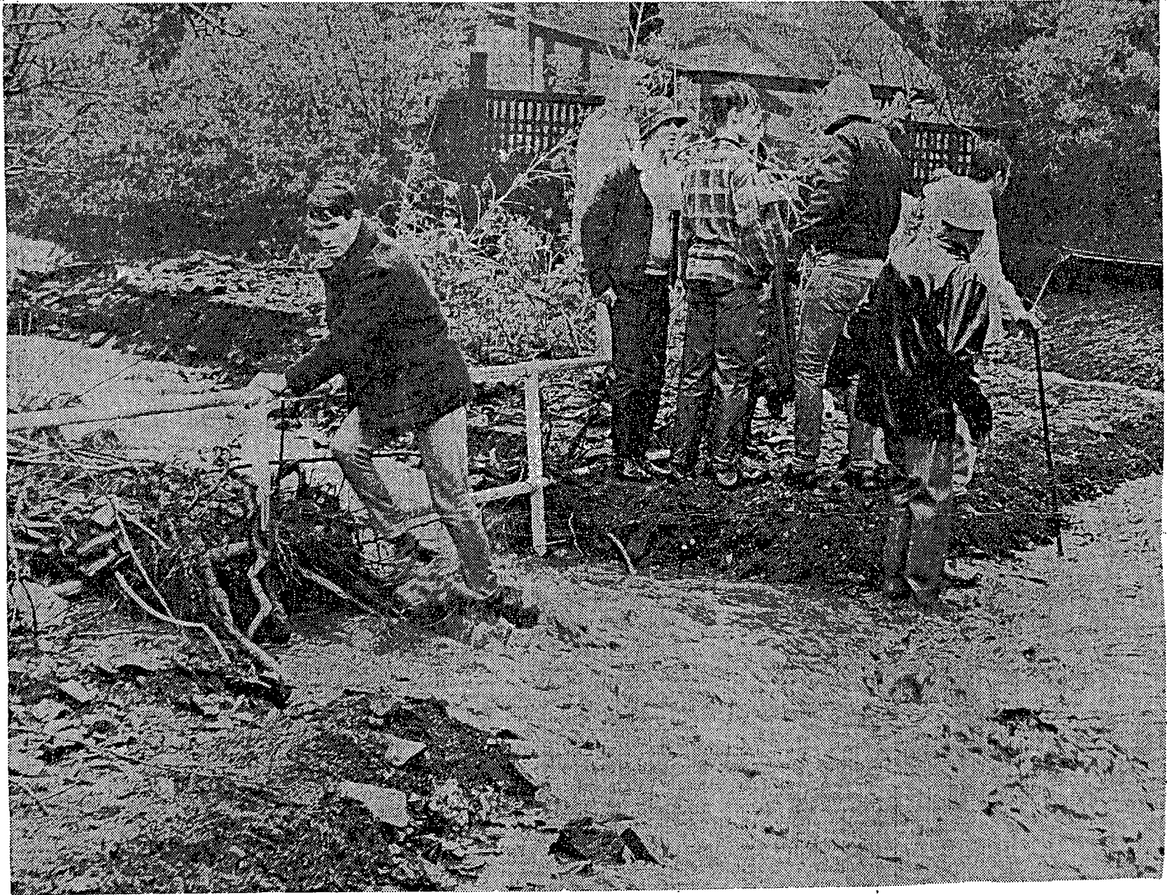
BRIDGE OUT —Flood waters overran and almost obliterated this Mandeville Canyon Road bridge making it hazardous to cross, but a similar bridge, below, which also crosses the creek, is high and dry two days after rain. There is still opposition from residents to install storm drain.
